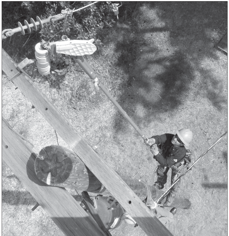
Clockwise from top left, Bill Richardson gives the thumbs up after his climb. Todd Niva secures Joe before he unbelts him. Jeff Speelman opens the cutout on the transformer to ensure power is disconnected before he continues up the pole to rescue Joe. Martin Taylor is all smiles after successfully rescuing Joe for another year.
